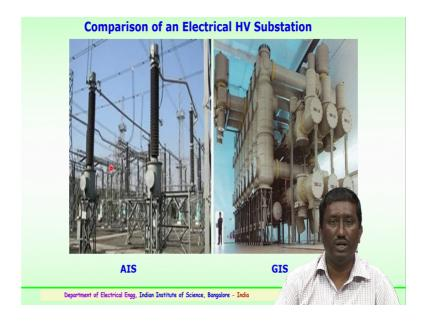
So, this is similar comparison of an electrical high voltage substation, you can see this air insulated substation which has exposed to the atmosphere lot of clearances and several complicated arrangements have to be carried out. Whereas for the gas insulator substation, it could be very compact and with the help of the sulfur hexafluoride gas it could be made compact.
