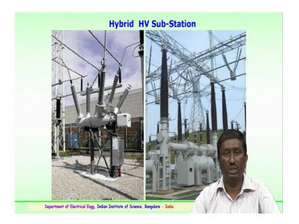
So this shows the comparison of a hybrid and hybrid high voltage substation, so gas insulated substation, air insulated we have seen. So, hybrid is a combination of the air insulated and the gas insulated; the important point being again it reduces the economy to a certain extant going in for full GIS could be more costly. So, in some of the cases transformers could be installed in the open yard, that is the outdoor and rest of the equipment could be gas insulated.
