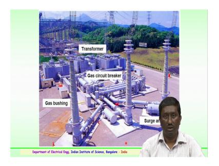
So, 1620 should be the residual voltage and the lightning impulse withstand voltage in case of transformer should be 1950kV and the gas insulated substation should be 2250; 2250 kilovolts are the specification for GIS. So, this is the typical gas insulated substation which is being seen here; it consists of a transformer, gas circuit breakers or the bushingm gas surge arresters. So, all are sulfur hexafluoride gas as a insulating media which reduces the entire cost and it is very very compact.
