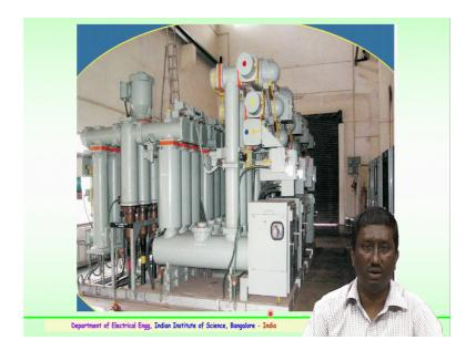
This is one of the example of a 400 kV GIS station, which also several switchgear and bus duct. So, a very compact size of 400kV typical substation will have several acres in the open air, here it is less than one-tenth of the required area in case of the air insulated substation.
