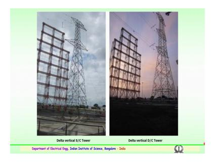
So, this is again a example of delta vertical single circuit tower here, this is again delta vertical arrangement for a double circuit tower. This is important the represent transmission system in the country is being witnessing a lot of advances are happening.
