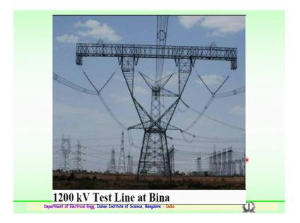
So, we are talking about 765kV transmission in the country, so now the power requirement has drastically gone up. So, lot of long distance transmission both at ultra high voltage AC and ultra high voltage DC lines are being constructed and several advantages in going for a long distance DC transmission. So, 800 kilovolts DC lines are being constructed across the country and DC and AC transmission of 1200 kV also is being thought for lost 4 to 5 years.
