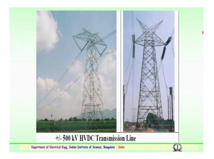
So, now coming to HVDC towers; there is a difference in case of a HVAC transmission line and HVDC transmission line. So, here the configuration varies with the load requirement; mechanical load changes here the conductors are employed or a different and the tower configuration also changes depending upon the clearances. So, these towers which are indicated here or for the high voltage DC transmission system; so, we have earlier looked into the AC transmission tower.
