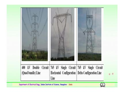
This shows a 400kV, a double circuit you can see double circuit again r Y b or 3 conductor in one arm; 3 more conductors has another set. So, this is entire thing a single circuit one more circuit double circuit; each phase again consisting of 4 conductor bundles. So, that is what quadruple bundle in; so, this entire 4 conductor bundle forms a single phase. You have two circuits here; this is again a tower configuration for 765kV single circuit with horizontal configuration as shown.
