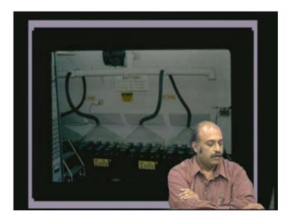
The photovoltaic array charges up this battery band and from this battery band it goes through a converter to supply the various loads as I showed or as I have told earlier in the block diagram.
