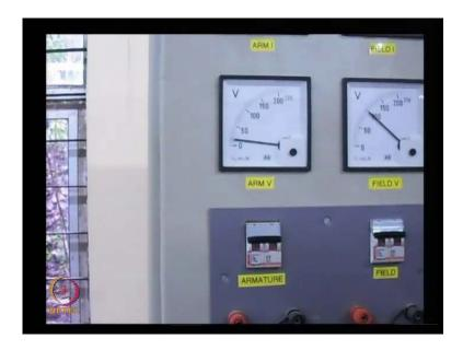
What I will do is the, I will disconnect the existing control rectifier and instead of that, I will connect the output the DC terminals of the diode rectifier to the synchronous synchronous machine field. So, that is what you have seeing here. So, the diode bridge is connected to the generator terminals on the AC side and the DC terminals are connected to the synchronous machine field winding.
