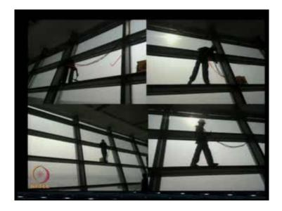
Now, we say the safety and the movement, and the work surface. Now, in this airport this person is cleaning the glass with different things and so the special tying things are provided here; so that he should not fall. Now here, which one is necessary to maintain this slope? If it is there, then how it will be cleaned? and like this way so means then We have to decide - which one is priority? What is actually required? Then keeping that fixed, other alternatives we have to take care.
