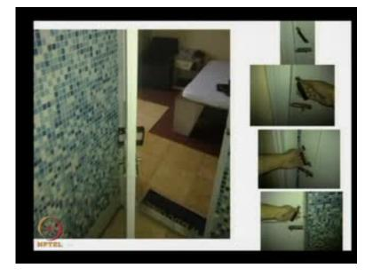
Now, again, something see the handle position, this area is inner side is the bathroom and outer side is the main room. So, that door itself here the handles put in a little diagonal way not in a horizontal or vertical because it will be easier to hold we cannot hold like this, we cannot hold like this; it is better to have a 45 degree angle at this position, so it gives that flexibility.
