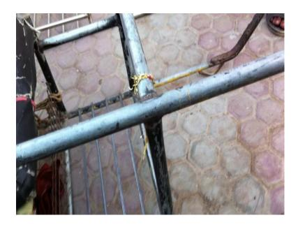
The GI water pipes Galvanized Iron and those pipes are very heavy, they are very thick.
