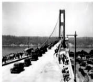
(a) Opening day of the Tacoma Narrows Bridge, Tacoma, Washington, July 1, 1940. The bridge was found to oscillate whenever the wind used to blow.
