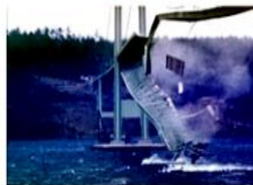
(b) The 1940 Tacoma Narrows Bridge collapsing in a 42 miles per hour (68 km/h) gust on November 7, 1940
