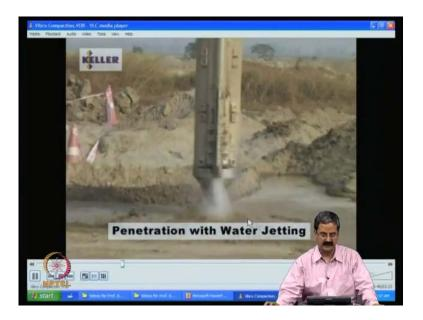
You can see jets. They have extension tubes. Coupling. It can be either water supply. So, they have an eccentric weight, they have a nose cone. Then you are trying to backfill in the same place the sand. You can see that it is a compacting.
