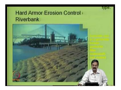
So, people may try to provide you know some sort of erosion control measures and river banks like this. In fact, say this is a concrete cast in a geotextile form. Geotextile filter is provided of course, it is not visible. (Refer Slide Time: 38:34)
