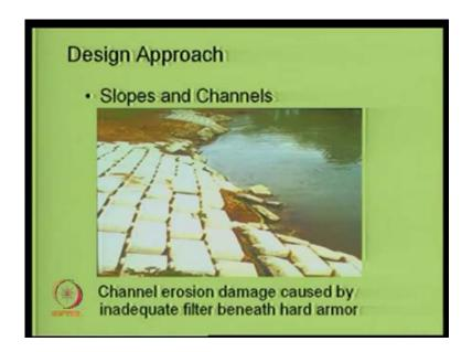
One can have and this is also another type of armoring in fact but then here the problem was that it is not the conditions are not cleared, that design was not good and maybe there is no connection between the two panels and if one panel comes out the all rest of that materials come out.
