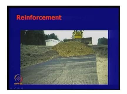
Reinforcement, in the case of roads, it can be done like this; where you have a granular sub-base material, you know; you have a sub-base material, and then you properly cover it and put a geogrid like what you have here. And, put the backfill soil or whatever is the sub grade material, sub-base material, and then role that, and then you have a very good properties.
