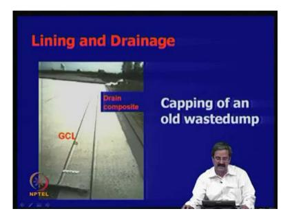
This is actually a lining and drainage applications here; what are you trying to do is that, capping of an old waste dump. Waste dump, say for example, now in India also we have lot of waste dumps. The count is not easy you know; there are so many waste dumps and we should see that the odors, the gases or whatever is that, the problem because of that should not be to the nearby public.
