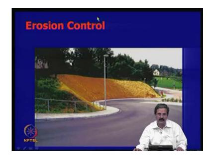
This is actually an erosion control mat here, you know; one can have a geotextile coir material and all that. This you can see that, as a slope is very nicely finished.
