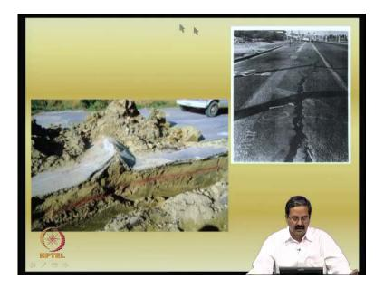
These are some typical failures that one can see. See, you can see a heave here, you can see very clearly a heave of the pavement you know, because the, you can see, that you know when the expansive soil is subjected to alternate wetting and drying and definitely, when there are some places where there could be more changes than the rest like...
