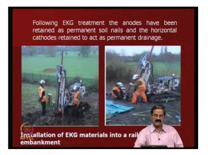
This is what they have been doing. Following E K G treatment the anodes have been retained as permanent soil nails and the horizontal cathodes retained to act as permanent drainage. It is very interesting. You can see that water is getting collected from the cathode. So, let it be act as a drainage in the slope. And there is a nails here put as anodes or the steel. Let it act as nails. It is nice. So, this is very interesting arrangement.
