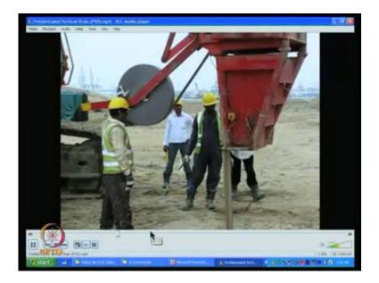
I will just show you this particular video in which you can see that this is actually prefabricated vertical drain. I was just mentioning in the last class, we have a sand drain in the olden days and we have now a PVD. Actually, the design is not very different, but the rate of construction of this is very fast like you know 10 meters it can go in a few minutes time.
