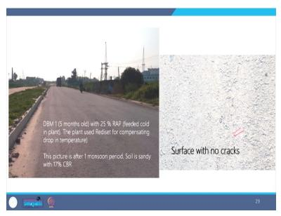
Well these are some pictures taken from one of the section where they constructed a DBM mix dense bituminous macadam, a binder course used in India with 25 percent RAP and this was feeded cold
