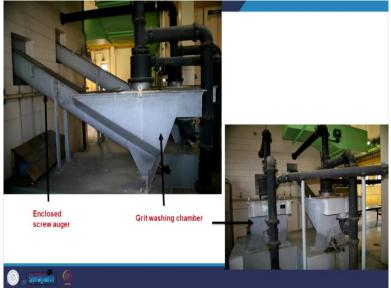
For example, from preliminary treatment we have the screw auger and then the grid washing chamber out here, let us look at what the grid looks like.
