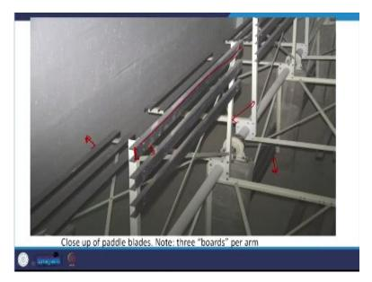
We have or we were looking at this particular aspect we were designing a paddle flocculators. Paddle, what are we talking about? These are paddle flocculators., we will have to look at the aspects such as the spacing between each; the width, the length, spacing between these and spacing from here to the wall, spacing from here to the bottom. These aspects you have to decide.
