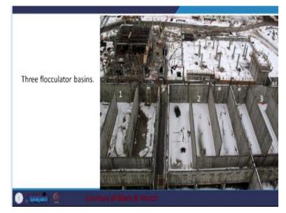
So, 3 flocculator basins. So, you can see them one here, 2 and 3. These are baffled type, , not baffle I think, these are not baffle type. Both baffle and with respect to the horizontal shaft mixing.
