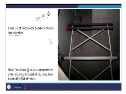
So, at the end, though, close up of flocculator paddle wheel, in the last chamber at the end, when the water is about to exit, to reduce the G in the last compartment, there are now only 2 instead of the usual 3. And in general, , you are going to have multiple compartments it is not going to be only one compartment with uniform level of mixing. So, initially relatively higher G may be 50 and then maybe 30 and then maybe 15.
