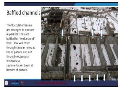
So, baffle channels let us see. The flocculator basins are arranged to operate in parallel, all 3 are parallel. They are baffled for end around. They are going to end and around. Flow will enter through the circular holes at the top of the picture and exit through the rectangular windows to sedimentation basin at the bottom of the picture. You can see this. Flow is coming through here; water will come this way and end and around and then it will exit here.
