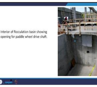
Interior of flocculation basin showing opening for paddle wheel drive. So, paddle wheel drive shaft this is what so, you have the opening for the paddle wheel drive shaft.
