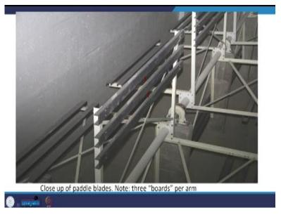
So, here, we see that there are 3 boards per arm, as I mentioned, the distance between the boards, pedal, is the term that encompasses all this setup and then the width and the length, these are the aspects we are going to look at. So, this is going to go over and above and over and above that how it is going to keep mixing.
