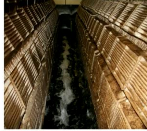
b) RBC with wastewater flow
