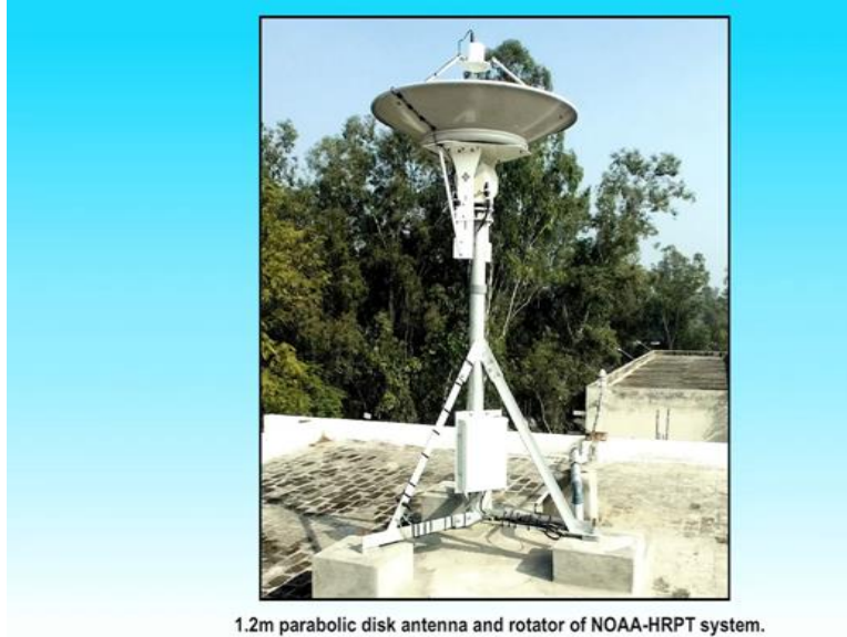
1.2m parabolic disk antenna and rotator of NOAA-HRPT system.
