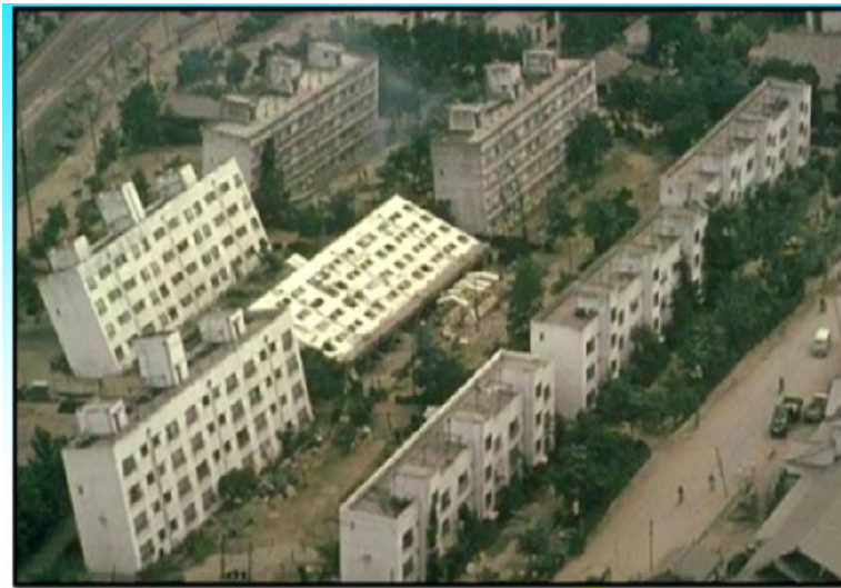
Some effects of liquefaction during the 1964 Niigata earthquake
