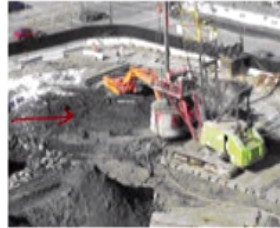
In-Situ Treatment Using Shallow Soil Mixing Method at Former MGP Site
