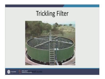
This is a trickling filter. So, in trickling filter, you have these pipes. These two pipes, if you can see carefully is your trickling filter and this bed is you filter, and these pipes are throwing the supernatant from primary clarifier. So, this is your waste water that has already undergone screening, grit removal and primary settlement and then this is thrown on this filter and this means that my bio films are going in this filter and what trickles out here is your treated water.
