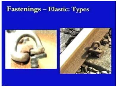
This is one photograph where the pandrol clip has been shown and this is another one where we can easily see that the shape of the thing which is provided at the bottom through which the clip is moving is like this and there is plate is being provided here and
