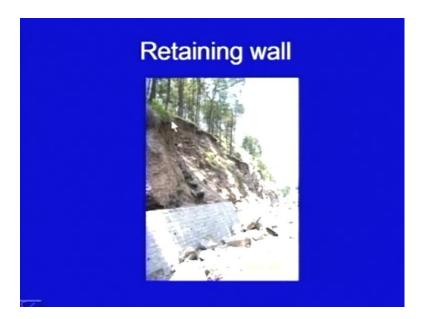
Here is an example, this is a slope here which is having retaining wall, this is the road on the side and this slope. This retaining wall is still under construction and this retaining wall is, is being constructed to retain this slope.
