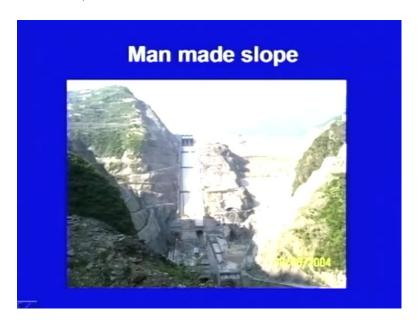
Here is another example of a man made structure, it is a dam here you can see it this is the downstream side of an earth and rock filled dam, upstream side is above that, water will be storing, water will be stored on the upstream side, a reservoir will be formed there and water will be exerting pressure on this dam. It will be seeping through it and the seepage pressure will also be acting on the dam body, inside the dam body, so here the stability of this particular structure is our concern.
