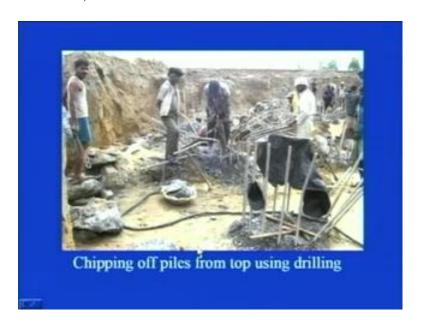
Now, how do you chip off the piles, see once the concreting is done and we really go for m 30 grade of concrete. So, and if the compaction has been done properly it becomes really difficult to chip off the concrete from that particular pile. So, with the help of this drilling machine, they just chip off that particular concrete, you must be wondering, that first we completed the pile at 30 meter and now we are chipping off this particular material from the top.
