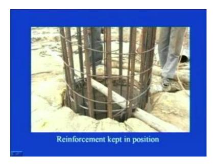
Then, as I told you that in one go you cannot lower this reinforcement, so you see to get this reinforcement cage, in position what is the kind of arrangement, that usually at site they go for, it is like a bamboo this thing, slab kind of a thing. They just place it in this bore hole and then you can see that they have made, it rested with the help of this lateral reinforcement, what are vertical reinforcement bar, we are main reinforcement.
