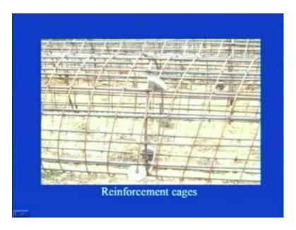
Then, you can see here, that particular reinforcement cage is lying, see these are longitudinal reinforcement, these are the, this is the particular rig, which is your lateral reinforcement and these are your ties. To bind this vertical parts, in position, then you can see there is a slab sort of cylindrical kind of a thing with a hole in between, you can see here in this one.
