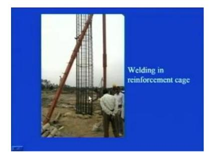
You see here, this is the bamboo that you are seeing with the help of which the reinforcement has been kept in position and you can see here that this particular labour is welding here. So, you see, this was up till this one, there was one reinforcement cage; some most of the portion has been lowered into the bore hole. However, with the help of this rig, another reinforcement cage has been lowered to the extent that, this particular worker is welding it.
