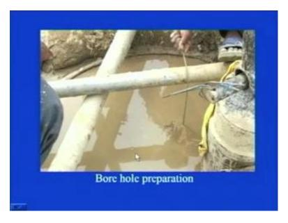
Then, in that was the case of driven piles, in case of bored piles, first you have to prepare the bore hole and then let us say the soil you have to go for say 25 to 30 meter pile. So, for that much depth of the pile, when you prepare the bore hole you have to make sure that the wall of the bore hole they should not collapse. So, for that you have to provide either some temporary or permanent measure to stabilise the walls of bore hole.
