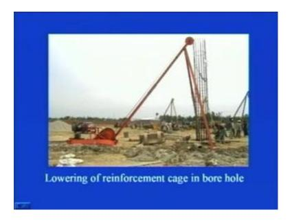
Then lowering of reinforcement cage in bore hole, see if you are going for 30 meter long pile, then the length of the reinforcement cage will be of that order and becomes like these are all steel bars and there you can see here this circular ones, rounded ones, they are ties, which tie these vertical main reinforcement of the pile. So, while lowering it down you see at a stretch you really cannot prepare a reinforcement cage of 30 meter and in one go you really cannot lower it down.
