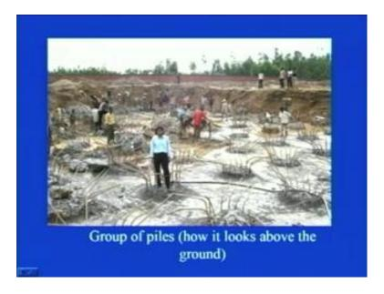
Then, this is another view, you see here that all the piles they have chipped off the concrete from the top and they have cleaned it and this is how I mean all the piles, you have the large area, lot of many number of piles are there. Some are being cleaned and some are there in the process of that chipping off and then cleaning of the concrete.
