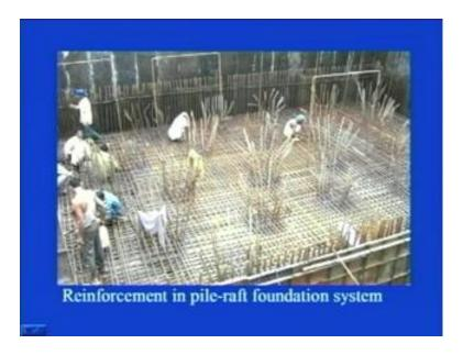
As, I was telling you, that this is what is this vertical bars, they which are visible here in this particular picture, they are the main reinforcement of the pile. And, this is the grid, which you are seeing this one, you can see that this is the particular grid; that is for the raft.
