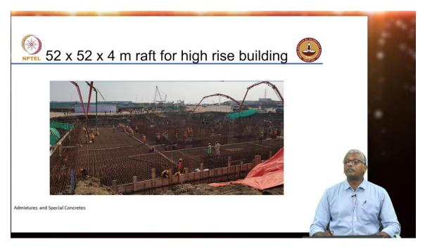
So, we were talking about the fact that the entire concreting operation was taken up by the means of 6 boom placers and 1 concrete pump so that the entire segment could be filled up in stages which were uniform with respect to the layer height throughout the 50 meter dimension of the member and then thermocouples were placed at different locations to get an estimate of the temperature rise.
