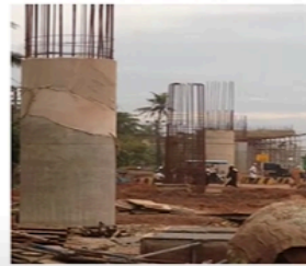
Construction of an elevated, coastal highway bridge
