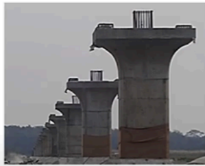
Construction of a river crossing bridge
