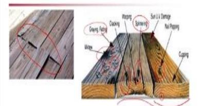
Now damage due to shrinkage, so you can see here on the left image that there is a pop-out different type of you know if you have been to places where Timber is used for flooring at etc. You will see this kind of problem because of the warping etc. So you can see that the right-side picture kind of shows the different types of problems that are experienced in such structures.
