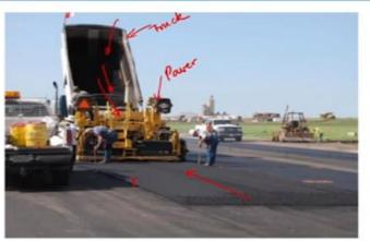
What is been shown here is the laying of the asphalt concrete. So, you have this instrument which is called paver. This is a paver truck, basically. So, what it does is it has this hopper which carries the asphalt concrete inside. If you are mixing it at asphalt concrete centralized plant, so you need this paver to actually bring that materials to the job site. So, you mix it somewhere and bring the material.
