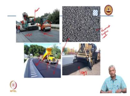
Again, I will show you that. Here you have the truck which has a tilting back which discharges the material into this paver. The paver is rolling out a thin strip and the roller is compacting, the pavement in that direction. This is the mechanized way of constructing roadway pavement. Again, another picture of the truck with more clarity where you can see the tilting back basically which is discharging the material and there we have the paver on this side.
