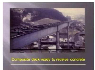
I can show you these are the composite decks you might have seen this today; the NHAI proposes many of these steel concrete composite bridges to span over the railway bridges; what is the reason? Because I can quickly launch, there is no blockage of traffic either train or road. So the columns are erected over the columns; we go and insert our beams, and you can see here these beams will have what is called shear connectors, and these are all braces.
