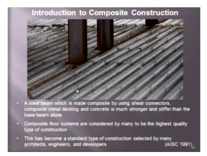
Now, this is the actual system; let us look; you can see here these are columns these are the primary beams. These are the secondary beam directions; we have just put the sheeting, and then we have put the stud you can see here.
