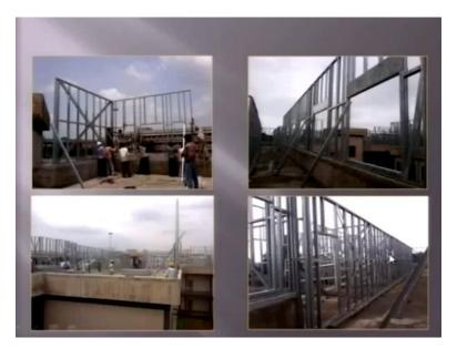
And this how the construction sequence was happening in this you can see here we are going to extend one floor what it is again on the circumferential wall this panel the wall cassette is fixed. And you can see this support are all temporary props till the top construction you can see here all the walls are ready in about a day or 2 then we put the roof cassettes and since the connections are very simple.
