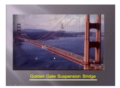
Of course, the suspension bridge with the cables we can see here you have the cable you have the suspenders and deck this is a classic example. We have a couple of examples of bridges in Goa, which are cable suspended bridges. However, the only thing as the technology and the car's competence, the engineers or contractors, start increasing by doing a couple of bridges. I think more bridges will be there.
