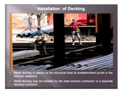
We can come and see here how the decks are placed. See, this is the primary beam between the column, so we have the secondary's just over the secondary beams we can put the sheeting. This sheeting can be made to any length because the rolling is done on the site we got a large coil. So we can load it quite nicely on the secondary beams, and after this, the studs are driven. And the studs, or you can see here the studs are driven on the secondary beam; after that, it is ready for concreting.
