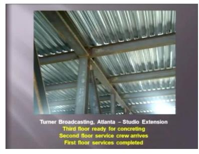
So this was a very good case for me present you can see here this I have just taken a photograph on the third floor that means the next day was the concreting. So you can see in the third floor you can see the main steel beams you get. The secondary is on which we are putting a steel deck sheet which has got corrugations to give us the moment of inertia. So we will have to put a small amount of reinforcement and then concrete on top.
