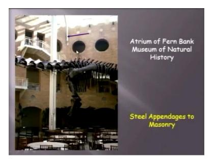
Not only that, you can see here that steel has been appended to their existing masonry as well. So this particular material is not standalone for use, but it will merge with masonry and quite nicely with concrete. And the usage, the steel say for example there is a large party hall, so you have a column-free space taken only by one particular central octagonal column. So this column supports a big truss work and truss work on top of it we put glass.
