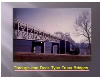
And again, this is an example you can see we have a deck bridge, which I mean immediately converted you are through a bridge. This is because of the navigational depth which is required. So many times, the structures are built not for the strength or the amount of load that comes; it is not about you know how many broad gauge trains are going to come. But it is navigational because we will you know abstract the navigational way possibly the fisherman or the fish species to migrate.
