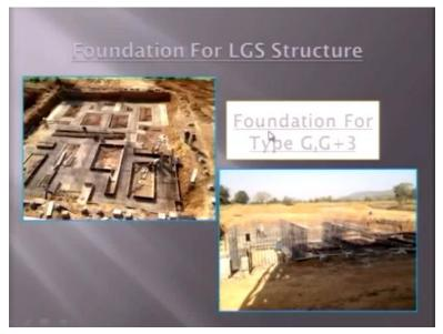
And there we have a very light foundation you can see here the foundation is just a simple spread is not very deep no piling. This foundation was for G+ 3.
