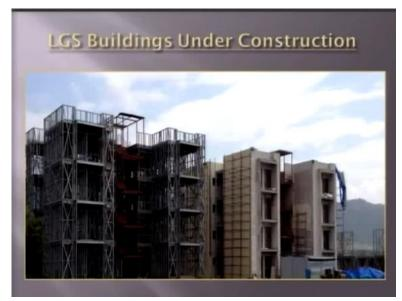
Now, this is the finished work you can see here; this is the work that is completed, and this is just going to be complete. You can see here the vertical staircase is of, I mean hot rolled steel, so you can see the hybrid structure all these ones which are galvanized cold-formed steel G+ 3. And this is a hot roll steel staircase; now this is almost entirely over, you can see all the side walls or CP boards.
