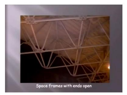
This is the steel space frame or a space roof that is architecturally synthesized; you can see on top of it steel sheeting. Amazingly, it has been integrated or synthesized with the existing concrete structure. So we can see steel, can you know to be a complementary material in very many situations, especially for beauty for aesthetics and construction time. So these space structures, which I will cover a little later.
