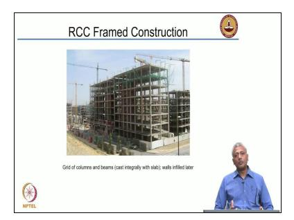
Now in most modern buildings, at least in the urban areas, we will see that people follow what is known as framed construction RCC framed construction. So here what we see that the columns, beams are coming on top of the slab; columns, beams, slabs are all made with reinforced concrete. So essentially, we make up a frame.
