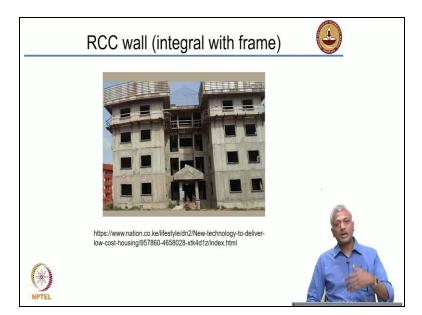
In some cases, if we come to a more modern type of construction, the wall itself is reinforced concrete. And many of fast track rapid housing construction projects will see that the wall is also reinforced concrete. So what happens is that the entire segment of the wall in the column is cast integrally, and it continues to move up. Our formwork which is here continues to move up as we are completing this construction.
