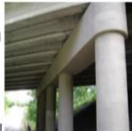
FRP wrapped bearing pedestal
