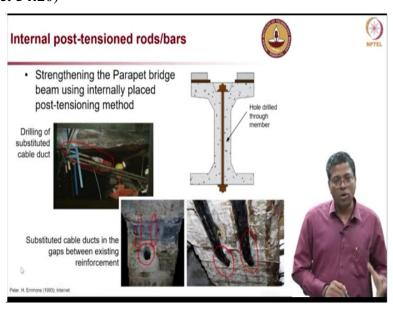
So I am going to show you couple of examples on some of these and then close the lecture. So strengthening the Parapet bridge using internally placed post-tensioning method, this is a case
