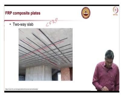
This is an example showing a two-way slab where you have these plates going and these are CFRP or carbon fiber reinforced plates. In a building structure, you can see they are going in both directions for two-way slab.
