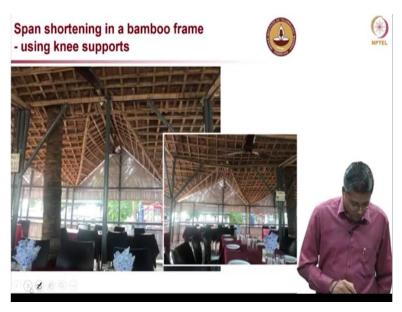
This is an example photograph, not a concrete structure here. It is just a bamboo structure, you can see there is an additional support given here. On the picture on the bottom right, you see a deflected bamboo beam. It is essentially a beam and that is supported by providing additional knee bracing and also sometimes this vertical column. So I just thought of showing you this nice image, which I took it in one of the restaurants in Gujarat.
