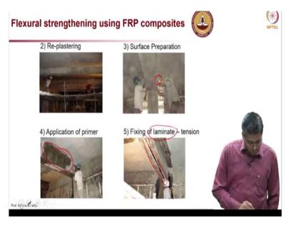
And then new plastering material was applied or re-plastered and then cleaned, the surface of the plastered surface was cleaned so that the chemicals or the primer and then can be glued well. So after the surface preparation, you can see a person cleaning it here, then to the cleaned surface this primer was applied and then the laminate. The stiff plate was glued to the bottom where the tension forces are acting, bottom most fiber.
