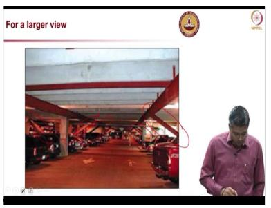
I am showing a zoom out image of this, so that you can see this is the bracing which we are talking about. You can see all these inclined elements; they are all the knee supports, which we are talking. And now when you talk about this, these knee supports, they are actually resting onto the columns which are visible and how the columns take these loads? That is also something needs to be considered and if they also need to be strengthened along with this work that also need to be done.
