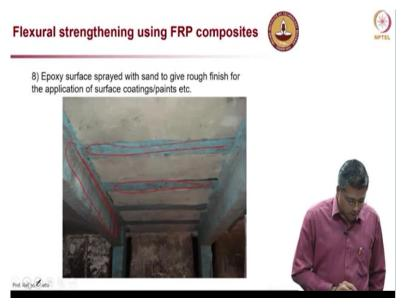
And then after that, before the chemical was dried, to have additional paintings and other coatings, you need a rough surface. For that purpose, sand was sprayed on the epoxy surface. So you can see here to get a rough surface finish, sand was sprayed so that other additional paintings, etc., can stick well or bond well to this surface. So that was the work, recent work on CFRP or strengthening using CFRP.
