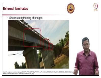
This is another example. Again you can see, the shear region is only the near support region. So this girder does not have any problem with the flexural resistance. The problem is mainly for the shear resistance, because shear cracks were probably observed in these elements like this and they wanted to fix that issue. So they provided this FRP laminates and that is only provided where the failure was observed not the entire bridge. So it is a good way of optimized use of repair materials.
