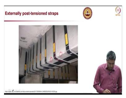
I am going to show another photograph. You can see here this beam is chamfered and this strap is nicely curved so it can easily take that load and give very good shear enhancement.
