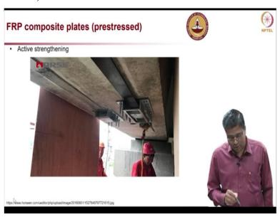
Now other typical application of this kind of plates is prestressed, which is an active system. Again you can see this girder here which is prestressed, you can see the marking of how the concrete surface was cleaned, you can see that in a bushing wheels marking on that. So cleaning is very important, otherwise they will not work very well. They are cleaned and then glue or whatever the adhesive is applied and then the carbon fiber reinforced polymer is placed and then it is prestressed.
