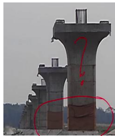
Construction of a river crossing bridge
