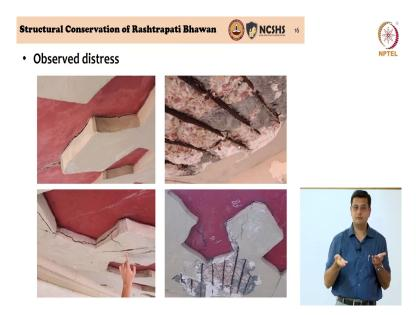
But the problem is today, that is the status of the sun shades; the sun shades at a height of about 50 feet and you have material that falls as you are walking in and out of the building. And you can imagine if a piece of lime concrete from a height of 50 feet where to hit anybody's head, you could actually have a fatal situation.
