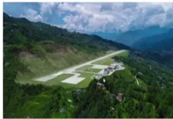
Pakyong Airport, Sikkim 2009-18. At 1400 m height; one of the tallest reinforced soil structures in the world;
