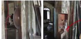
Unsuccessful extraction by saw cutting
