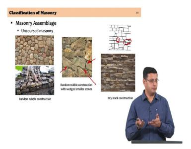
If I now move on from course, from units, masonry units and mortar which is the constituents to assembly, assemblage of masonry. Uncoursed masonry has been used in many of the existing masonry constructions. Random rubble construction is one of the uncoursed masonry constructions wall constructions where both in elevation and in cross section you would not see a pattern, it is totally free of regular courses and as I said, has a certain randomness to the entire construction.
