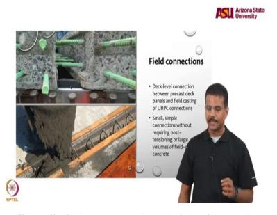
Ok field connections like I talked about, you can have deck level connections, connections at the deck level where the two panels of the deck are connected by UHPC or you can have the deck or the Girder connected to the support structure through UHPC, so multiple ways of doing it. The advantage of such extreme high strength is that the connections can be small and you are always better of doing smaller connections than larger connections because connections are the weak points.
