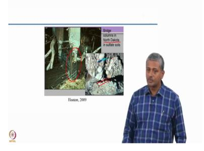
Again this is a example provided by Professor Doug Hooton from the US where these columns are standing in North Dakota in sulphate soils and you can see that almost all of the concrete in the cover zone is completely spalled you can see the pieces of concrete lying around, so much expansive stresses have been generated that you are spalling is tremendous in these columns.
