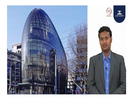
Because it need not be a square or rectangular it can be have a curved shape or any shapes you know it can have this. So, that is the speciality of the IGU you need not to be constrained about only one there are 2 dimension like rectangular square. It can be a cloud shaped or shape of the like you can see that they made a kind of a shell or we can say the egg kind of this, it can be done through glazing with the help of IGU.
