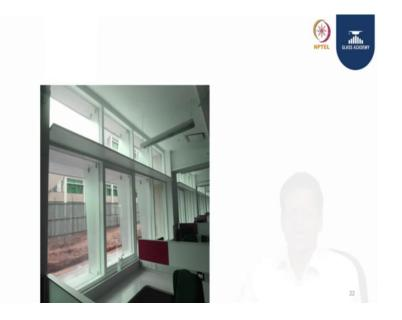
This is a typical balanced section where internal light shelf is given of around 2 feet, we have around 2.3 2.4 meter facade having day light pane. We have a vision glass, day light
