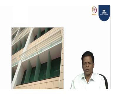
This again external view of a balanced facade having see the shape of the glass fin where it is a tapered. These are all data's simulating from sun path analysis. And the external shading element considered design as a combined unit where first 2 feet portion is designed as a solid, later we have aerofoil louver to this is to bring aesthetics to the building also.
