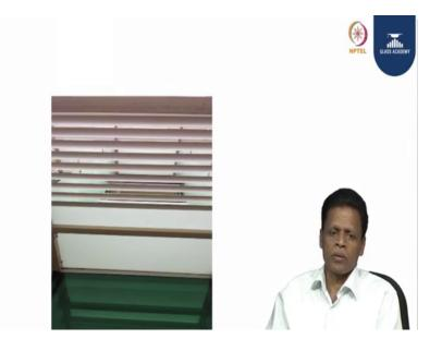
We have aerofoil louver again we have option of partly frosted glass and partly aerofoil louver.
