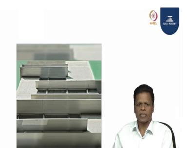
This here we can see lot of external shading elements are used chajjahs are used the here we used solid aluminium composite panel where the area having very bright sunny sun of the part of the countries, we can use the solid aluminium chajjahs here we used box sections in a loured manner to add aesthetic at the same time it will cut down the radiations up to certain extent. And through that vertical light will be given. So, that the facade externally facade will be properly lit.
