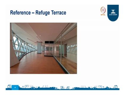
Here are some examples of how glass is being used in refuge terrace. So, you can see if you do not use a fire resistant glass again, the why do why does one need to use a fire resistant glass in refuge area is, because there is a possibility that the fire can spread from the area of occupancy to the place, where people are taking refuge. (Refer Slide Time: 18:23)
