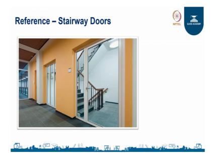
Here is another example of stairway door, in which you can see that a fire resistant glass is used in a fire resistance system. Again, if we do not use a fire resistant system in this place, there is a possibility that the fire could spread from the area of occupancy into the fire exit passage. So, when people are being evacuated through this areas, if there was a fire spread into this region into this area of evacuation, then it hinders the whole evacuation process.
