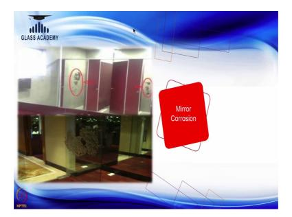
The first defect which is known as mirror corrosion, now why this mirror corrosion is happening is again because of incompatible adhesive. When I say incompatible adhesive it means the adhesive, which is being used to fix that glass was not compatible to the back paint.
