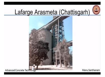
So the material then comes out and stored in the silos and finally dispatched.
