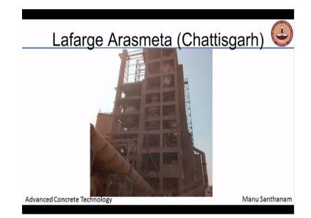
Now I do not know how clear this image is. This image is that of a preheater tower. Why is it called a preheater tower because there are several preheater modules connected to one another vertically. So you can see that this is nearly 8 to 9 storeys high and there will be at least 6 to 7 preheaters connected in series to one another so that the material gets thoroughly preheated, all the moisture is removed.
