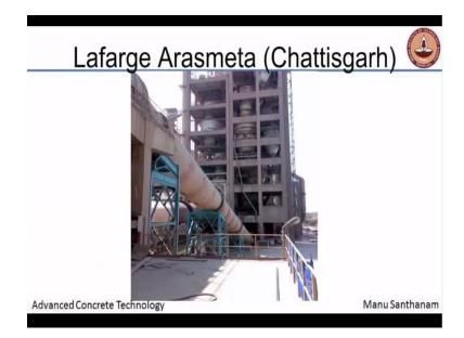
From the preheater tower, the materials come into rotary kiln but of course you see 2 different tubes here. The rotary kiln is here on this side, okay. This tube here is the heat recovery tube which is actually taking the heat from the cooling process back into the preheater. You see it is sloping the other way, so from the preheater the kiln has to slope in this direction. So this is the kiln which is sloping in this direction and I will have clearer picture of the kiln.
