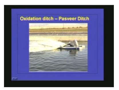
Here there will not be any sludge production or the sludge production is minimal and whatever the sludge is coming it is completely stabilized so we can discharge them into the sludge drying beds. This shows the photograph of an oxidation ditch.
