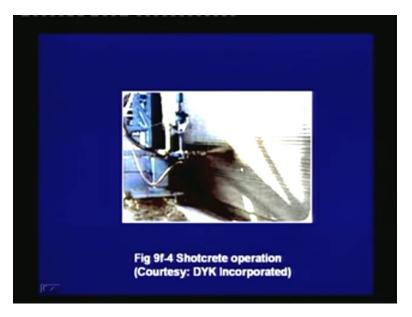
Next, a shotcrete machine is used to provide a coat of concrete over the prestressing strand, which checks for any corrosion of the prestressing tanks.
