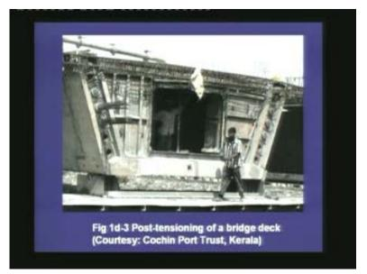
In a similar section after it has been post-tensioned, we can observe that the tendons are sticking out from the end blocks. Once the full post-tensioning operation is done in one duct, then the extra excess amount of the tendons is cut off, and the end anchorage block may be covered with grout so that it is not subjected to corrosion.
